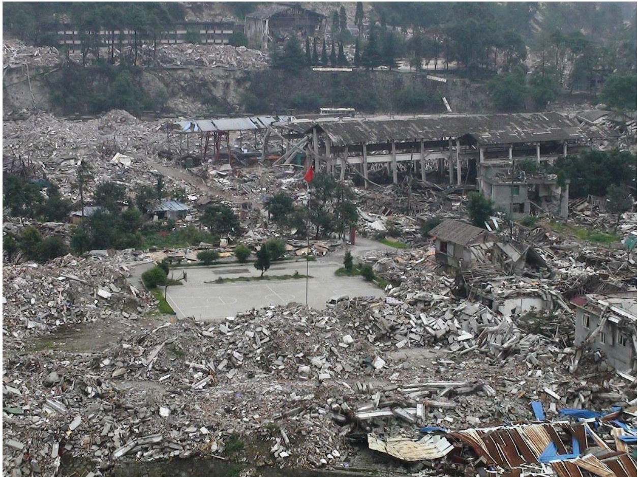
2008 Sichuan earthquake damage
